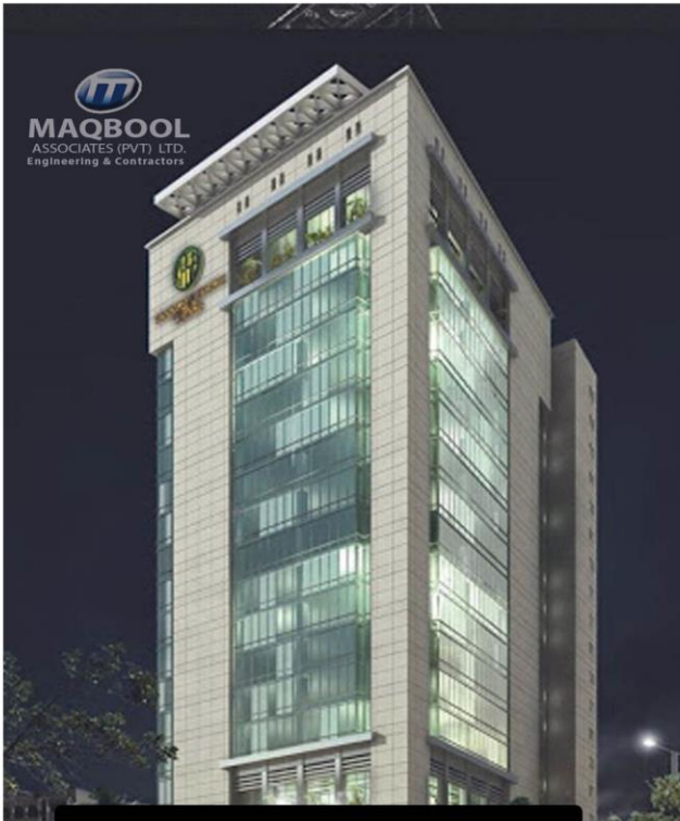
KASB Building Karachi
